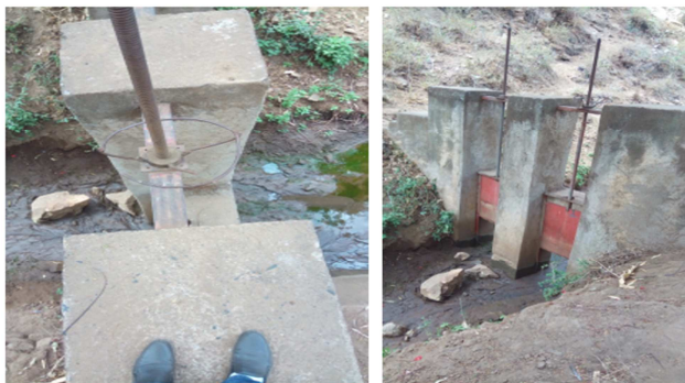
Figure 17. Malfunctioned flow regulator and present condition of the scheme.
