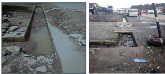
Figure 15. Storm water drainage system filling by solid waste and lack of clearance.
