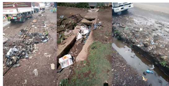
Figure 14. Dumping of solid waste in the storm water drainag.
